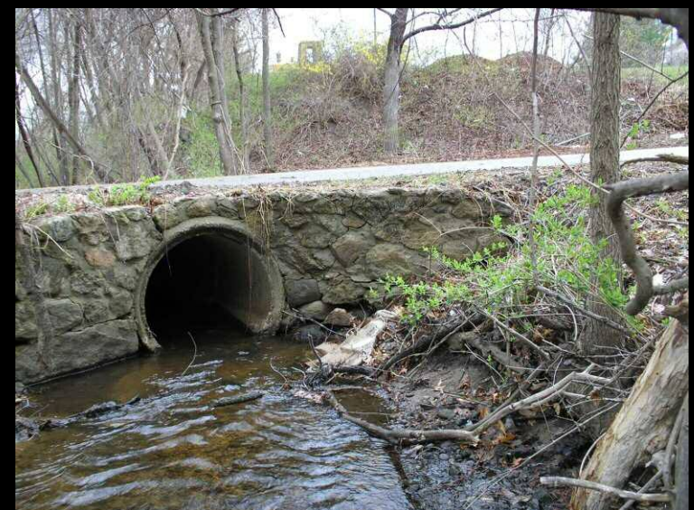
Wathen Road 36-inch culvert
