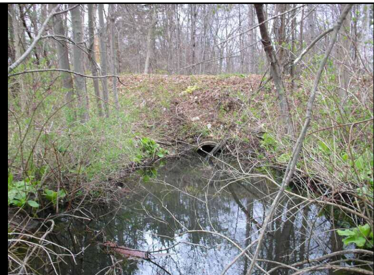
Eastman Avenue 36-inch culvert
