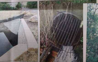
A new bridge and culvert give a clear path for McQuesten Brook to travel under Eastman Avenue in Bedford (Point 4 on map).
