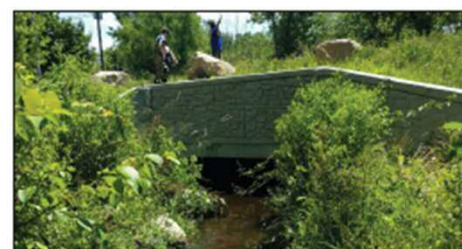
Figure 2. A new bridge crosses Eastman Avenue.
